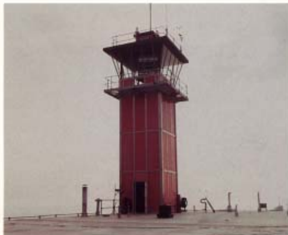
The light tower on Ambrose houses a 10-million-candle strobe that flashes white every 7\frac{1}{2} seconds (left). Time hangs heavily at the Ambrose Station for Coast Guardsman Paul Johnson on watch in the control room.
