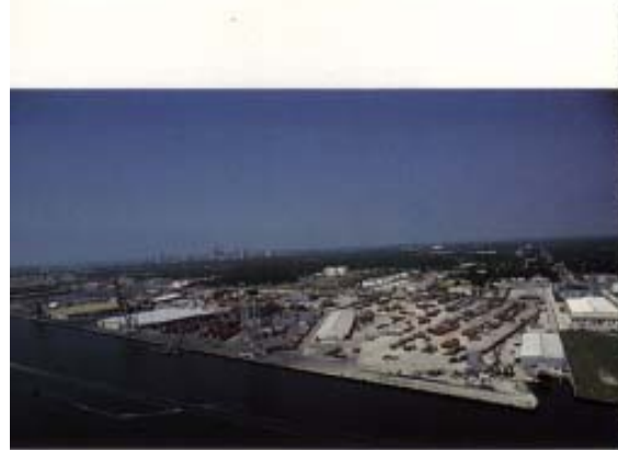
Talleyrand Marine Terminal
