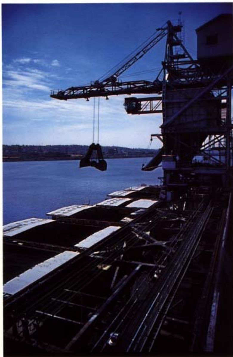
The Moran bulk Barge VIRGINIA , is unloaded by the crane at the Montaup Electric Company's power plant. HEIDE MORAN delivered the barge to the plant.
