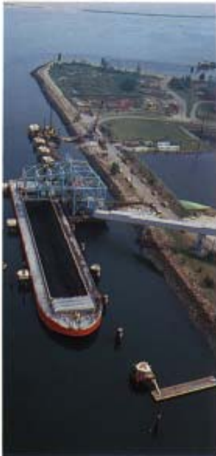
The barge BRIDGEPORT unloading at the United Illuminating Company's Bridgeport Station.
